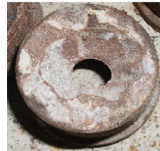
Fig. 5. Erosion failure of ash-blowing nozzle.
