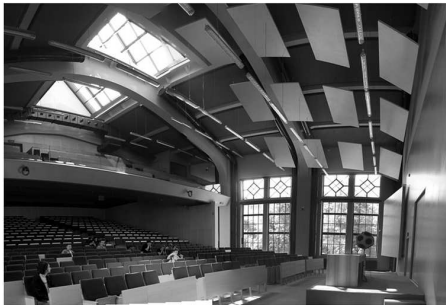
Fig. 1. Reflection panels in conference hall, AGH — University of Science and Technology, Cracow.
